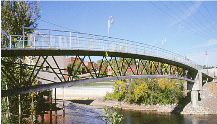
Fig. 4: Bridge made of self compacting concrete
